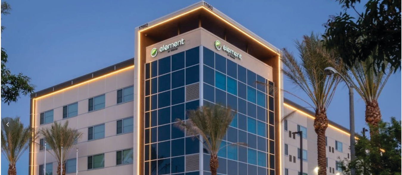
The ABR-owned hotel, Element Irvine, was intuitively constructed with an efficient use of space and a focus on sustainability.
